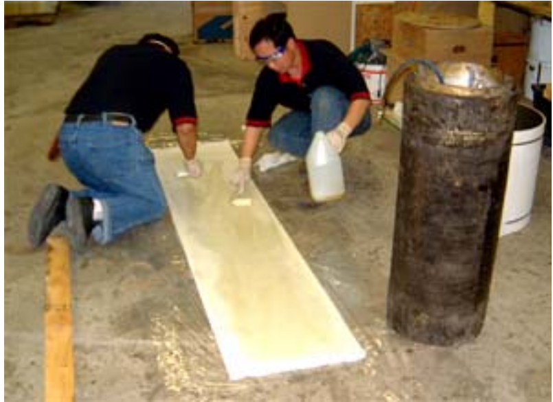
Fig. 5 - Spreading the Epoxy Grout
