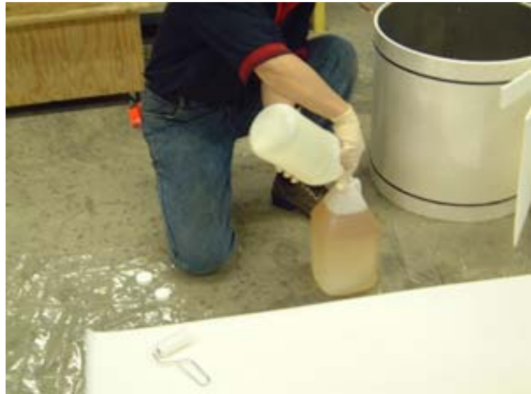
Fig. 4 - Mixing the Grout
